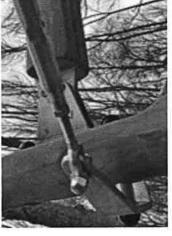
The hardware is made of stainless steel or galvanized steel to ensure durable connections with a high corrosion resistance.
